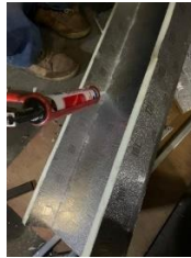
Gambar 7. Ducting aliran angin evaporator
