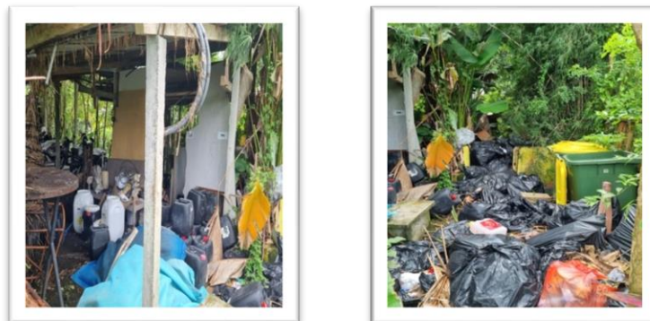
Figure 3. Condition of waste shelter at Dedary Kriyamaha Villas Ubud
