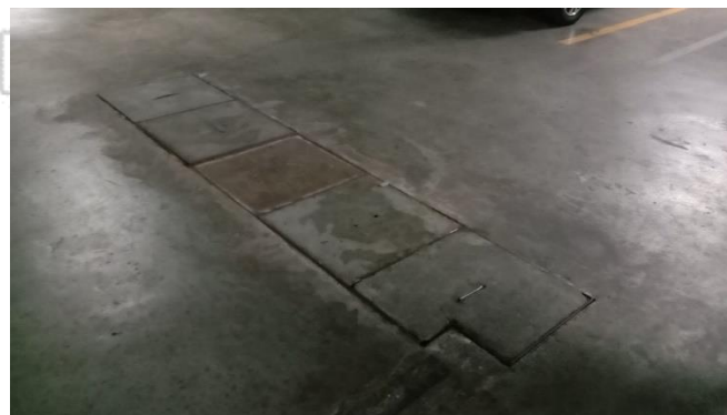
Figure 4. 22 Sewage treatment plant (STP)
