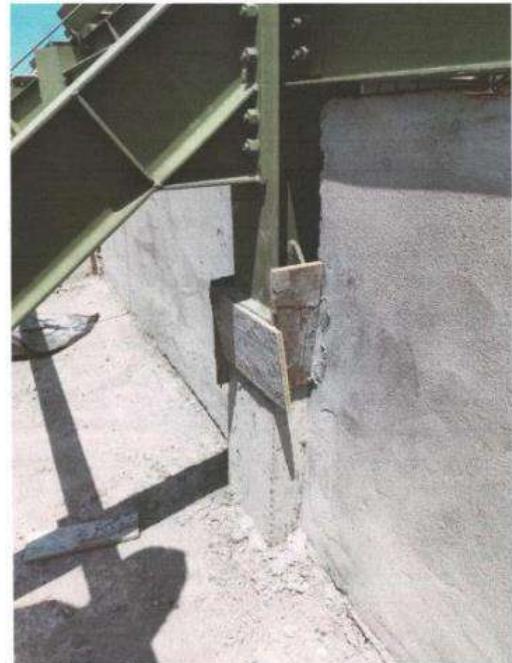
Kolom Lantai Atap (Atap 3)
