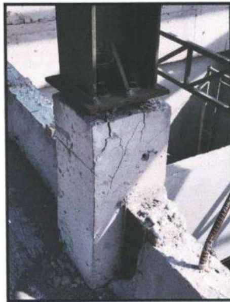
Kolom Lantai Atap (Atap 3)
