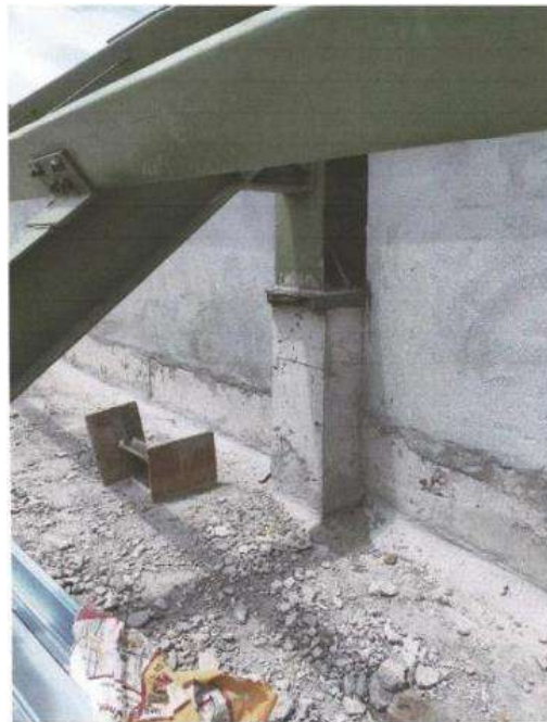
Kolom Lantai Atap (Atap 3)
