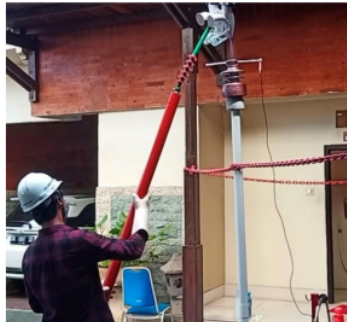
Figure 5: Online pedestal insulator washing.
