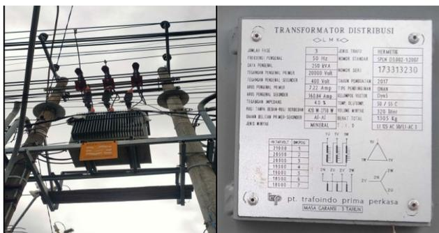
**Gambar 1.** (a) Gardu DB0575 (b) name plate transformator DB0575
