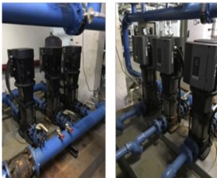
Gambar 5. Instalasi sistem suplai air bersih di Double-Six Luxury Hotel Seminyak
