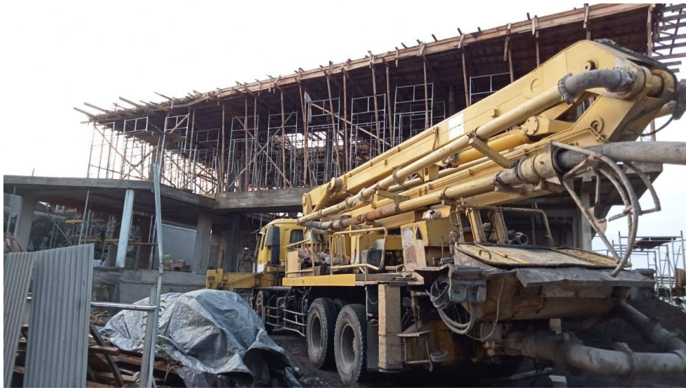
Dokumentasi concrete pump
