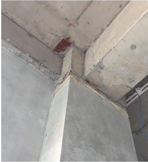
Sisa kayu, kawat, dan paku bekas bekisting plat as 7/I'
