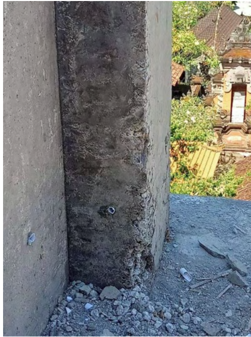
Bagian bawah kolom k1 as 10/K keropos
