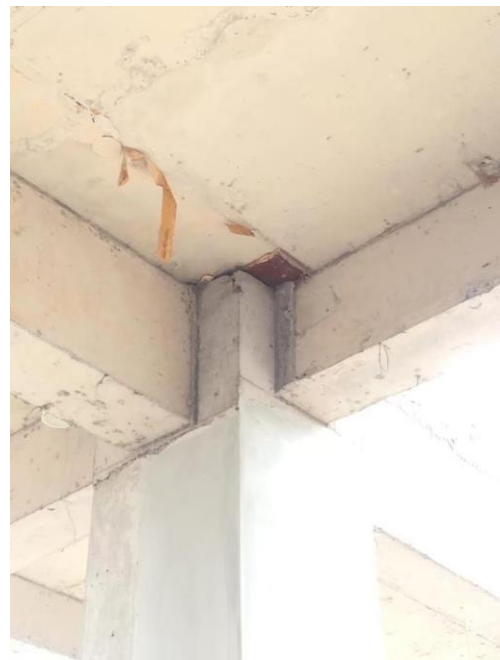
Sisa isolasi dan kayu bekas bekisting plat as 5-6/H-I
