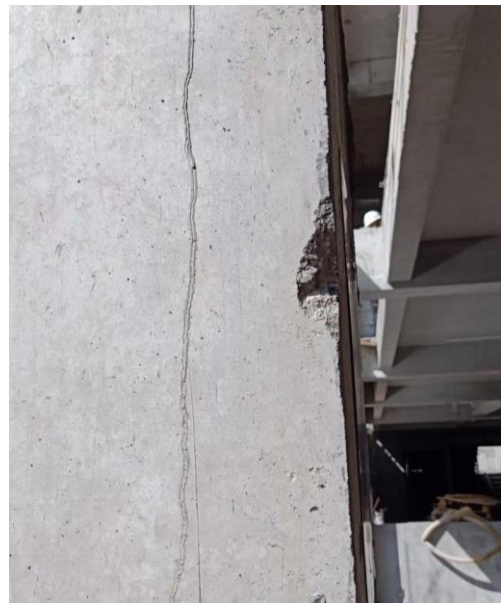
Bagian sudut kolom K1 as 5/H gompal
