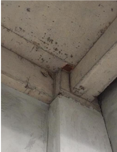
Sisa kayu bekas bekisting plat as 4-5/G-H
