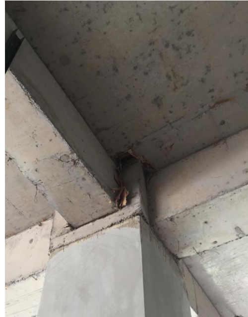
Sisa kayu bekas bekisting plat as 4/H
