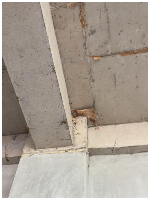
Sisa kayu, kawat, dan paku bekas bekisting plat as 7-8/J-K
