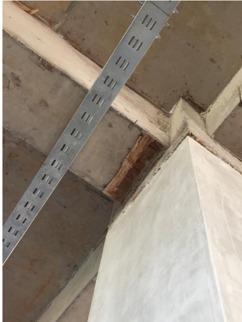
Sisa kayu dan paku bekisting balok B1 as 6/J-K
