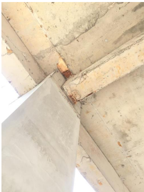
Sisa kayu dan kawat bekas bekisting balok B2 as 2-3/H
