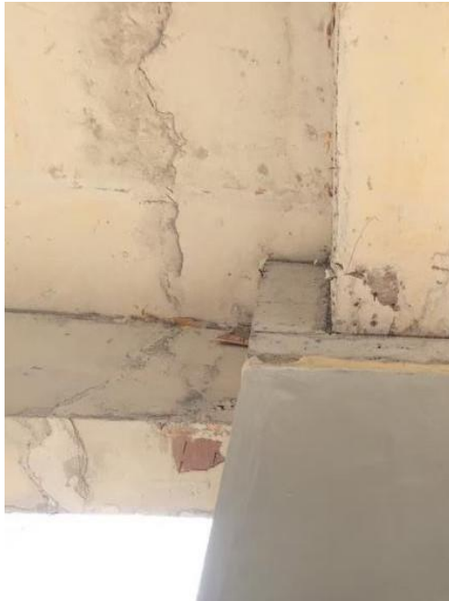
Sisa kayu bekisting balok B1 as 5/I-J
