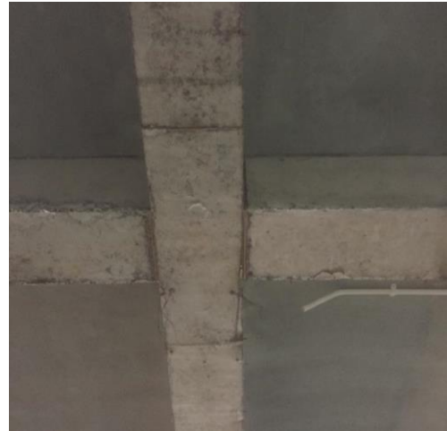
Sisa kayu dan kawat bekas bekisting balok B3 as 7-8/J-K
