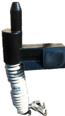
Gambar 9 Tekep Isolator Incoming Fuse Cut Out
