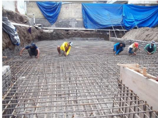
Gambar 2. 4 Pondasi rakit (raft foundation)
